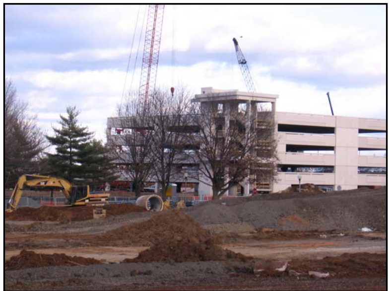
Figure 1. View of Parking Garage project from CI site
